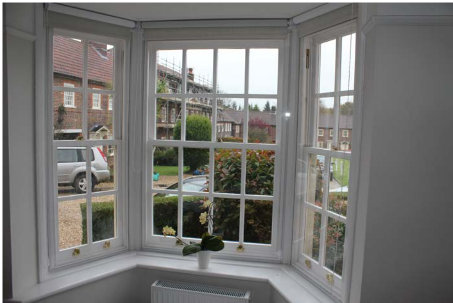
This is our lounge bay window with three acrylic panels in place
